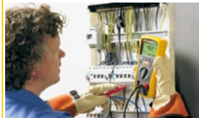
Insulation test at a distribution panel
